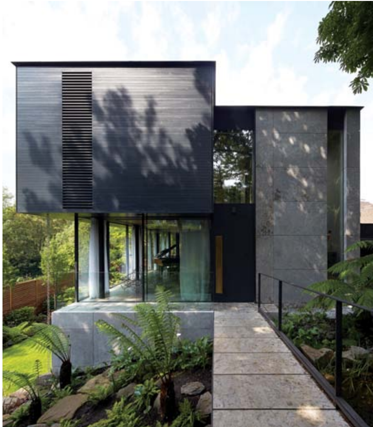
◀ Using a mixture of concrete, steel and timber for the structure, Stanton Williams (020 7880 6400; stantonwilliams.com) replaced a Fifties dwelling in north London with this three-storey house. It worked out cheaper than a prefabricated system, and took about two years to complete
