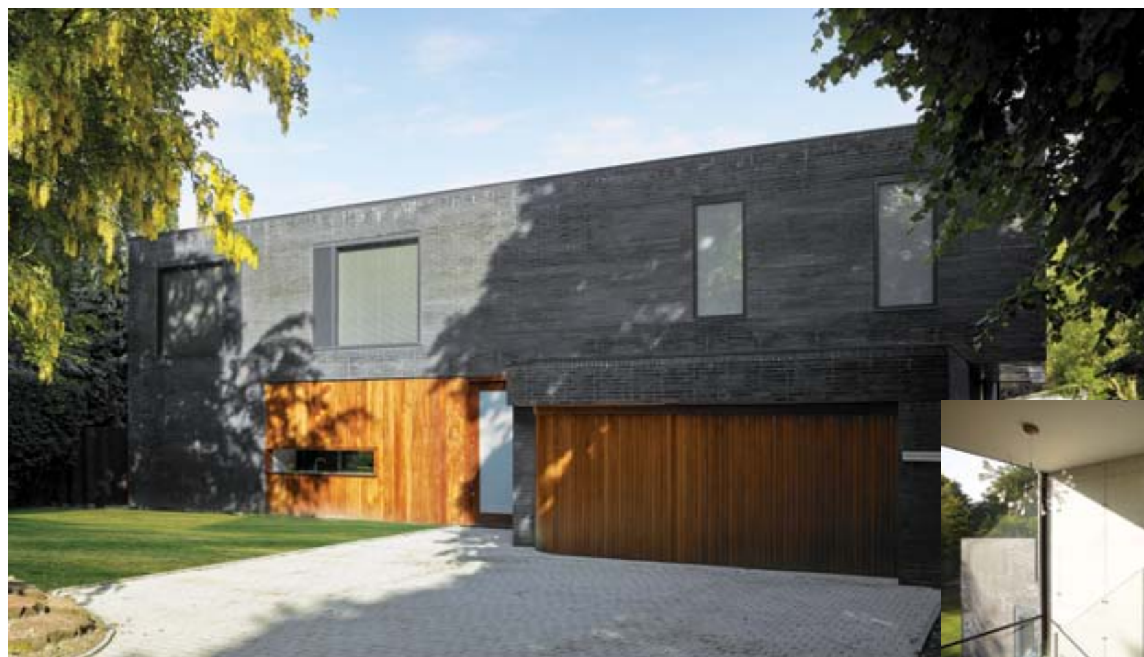
◀ A concrete frame and brick exterior skin was used for this house by Snook Architects (0151 707 0100; snookarchitects.com), which took 12 months to build at £1,250 per sqm (excluding land, kitchen, external works and fees). Concrete was chosen because of its natural heat storing properties, and was left exposed inside
